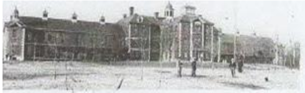
VGH – 1890 to 1948 when a new hospital was built
